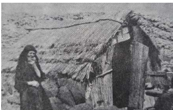
Figure 7. „Mlikar“ wooden structure with turf cladding (Mihić, 1985)
