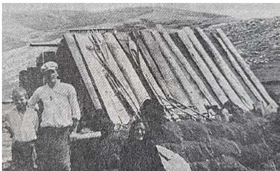
Figure 6. „Stan – koliba“ wooden structure with turf cladding (Mihić, 1985)
