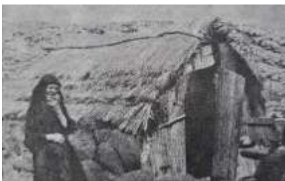
Figure 7. „Mlikar“ wooden structure with turf cladding (Mihić, 1985)
